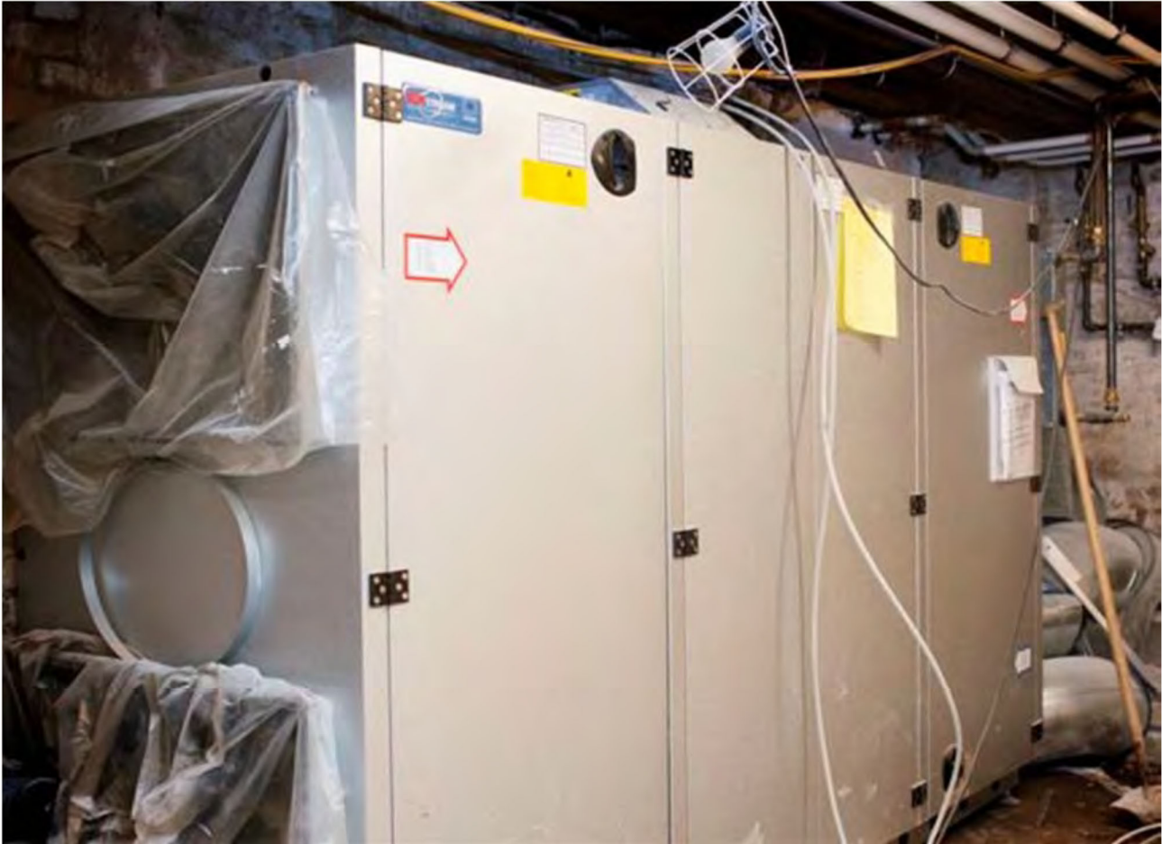
Fig. 1. Traditional central ventilation system.
